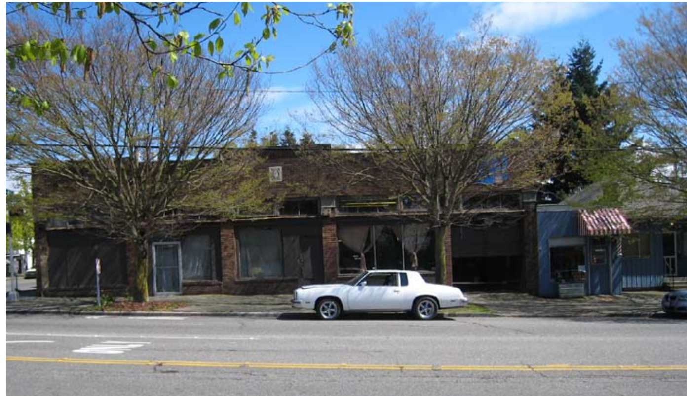
Large pedestrian-oriented storefront windows; durable building materials
