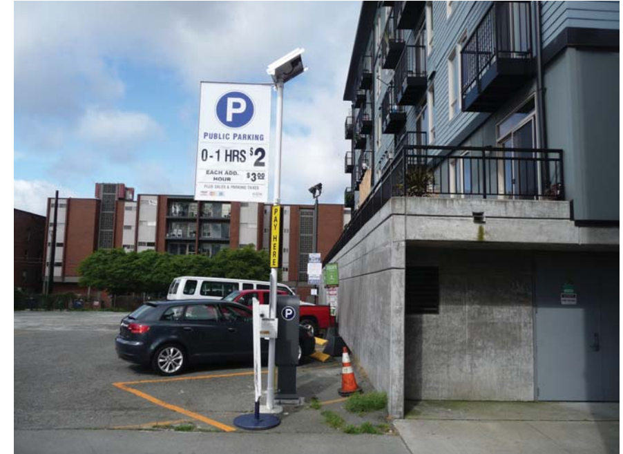
HEIGHTS APARTMENTS LOOKING WEST, CONCRETE WALL ALONG SITES NORTH PROPERTY LINE
