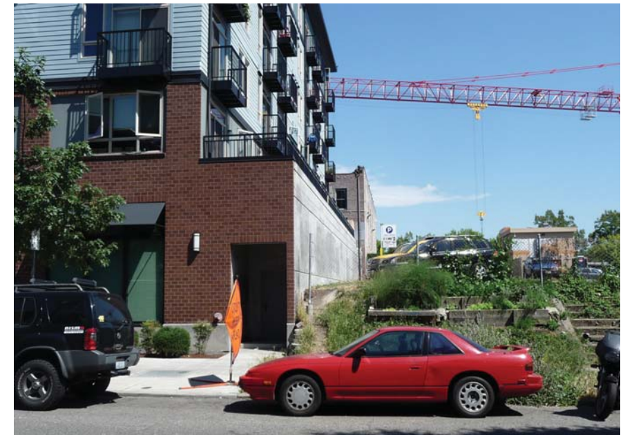
HEIGHTS APARTMENTS LOOKING EAST, CONCRETE WALL ALONG SITES NORTH PROPERTY LINE
