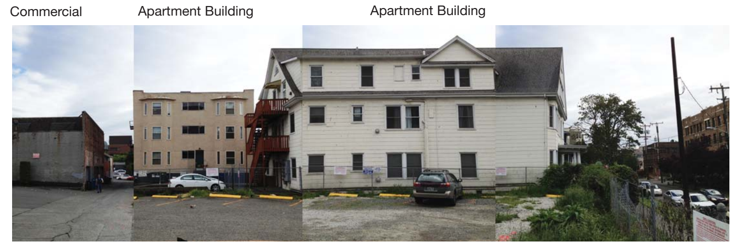
Alley ON SITE LOOKING SOUTH
