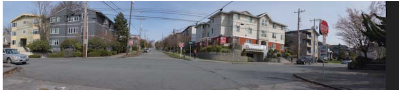
A 42ND STREET NE LOOKING NORTH
