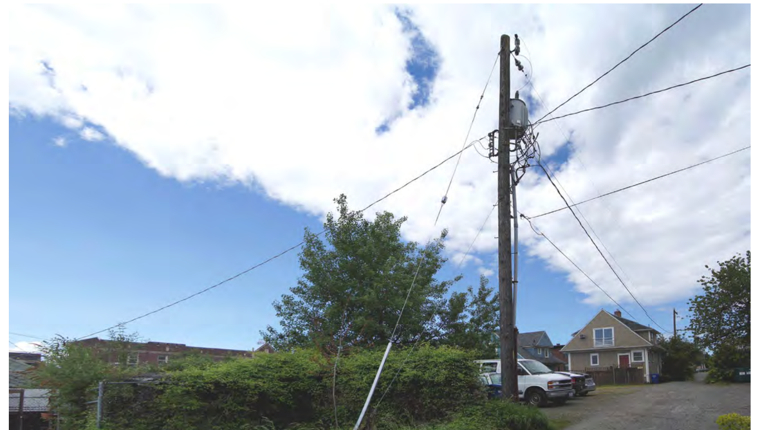
alley looking northeast
