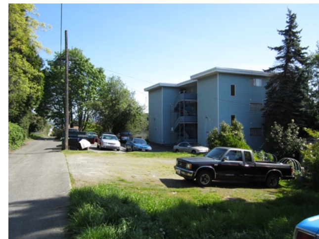
19 - ALLEY - LOOKING NORTH
