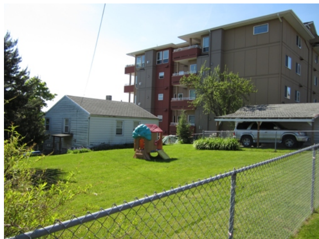
17 - ALLEY - LOOKING SOUTH
