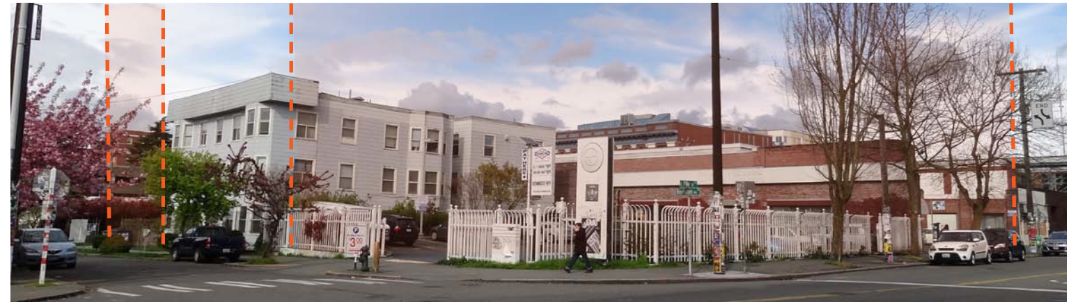
4. CORNER OF BOYLSTON AVENUE AND EAST PIKE STREET
