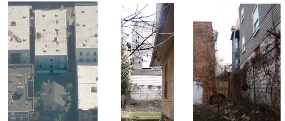
ADJACENT BUILDING - EAST PROPERTY
