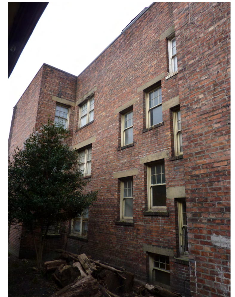
C) NORTH BUILDING FACADE - INSET AT PROPERTY LINE
