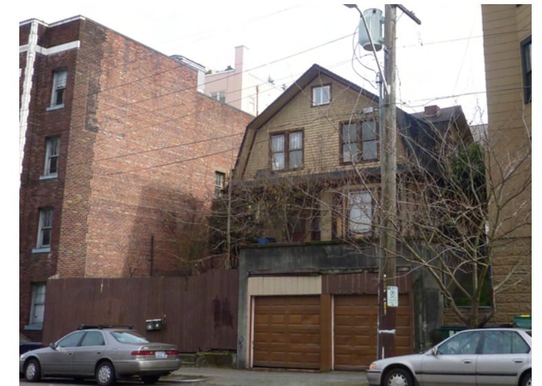
B) NORTH BUILDING FACADE
