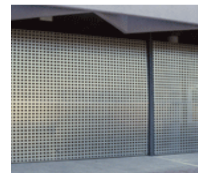
⑪ METAL GRATE OVERHEAD GARAGE DOOR
