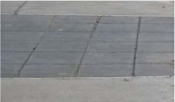
CIP Concrete Paving with Integral Color and Decorative Scoring
