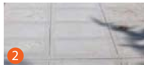
2'x2' CIP Concrete Sidewalk
