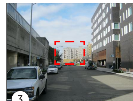
NE 41st St (Looking West)
