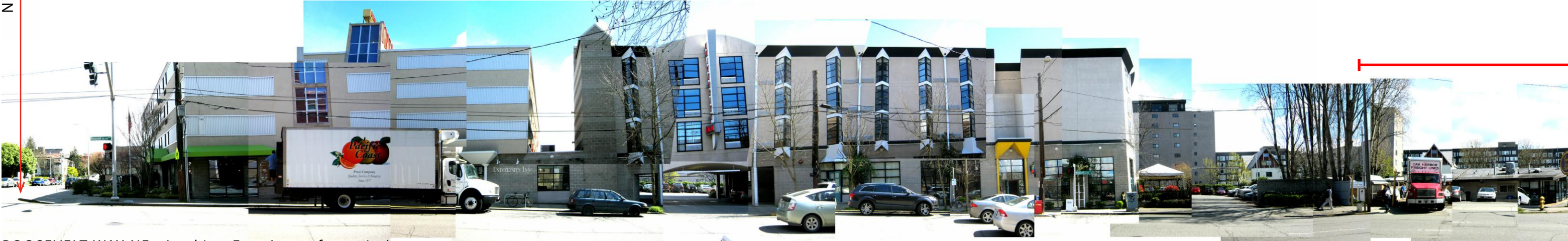
ROOSEVELT WAY NE - Looking East (away from site)
