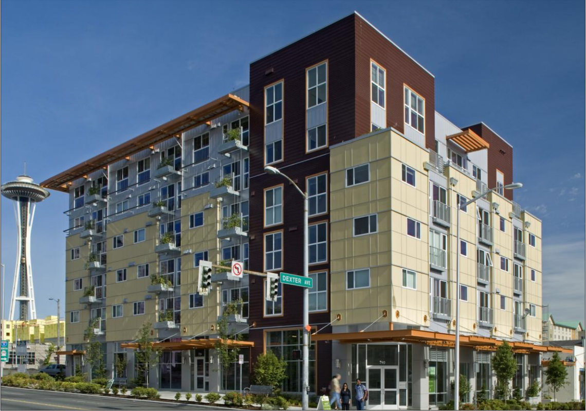
Borealis Apartments Runberg Architecture Group & Vulcan Real Estate
