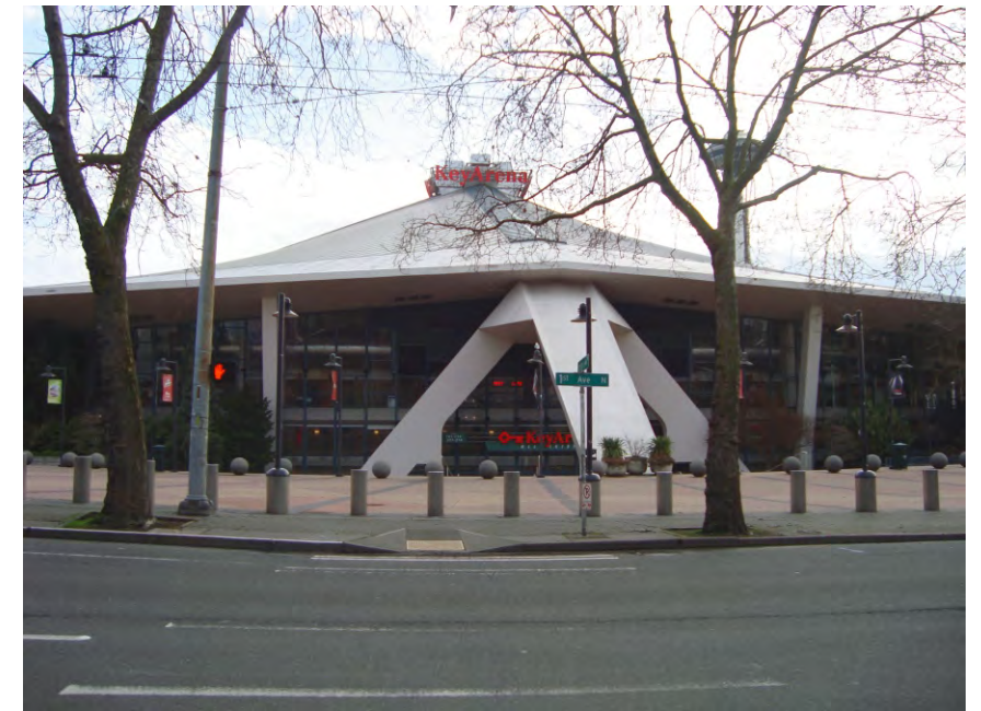
5 - W. HARRISON ST. - LOOKING EAST
