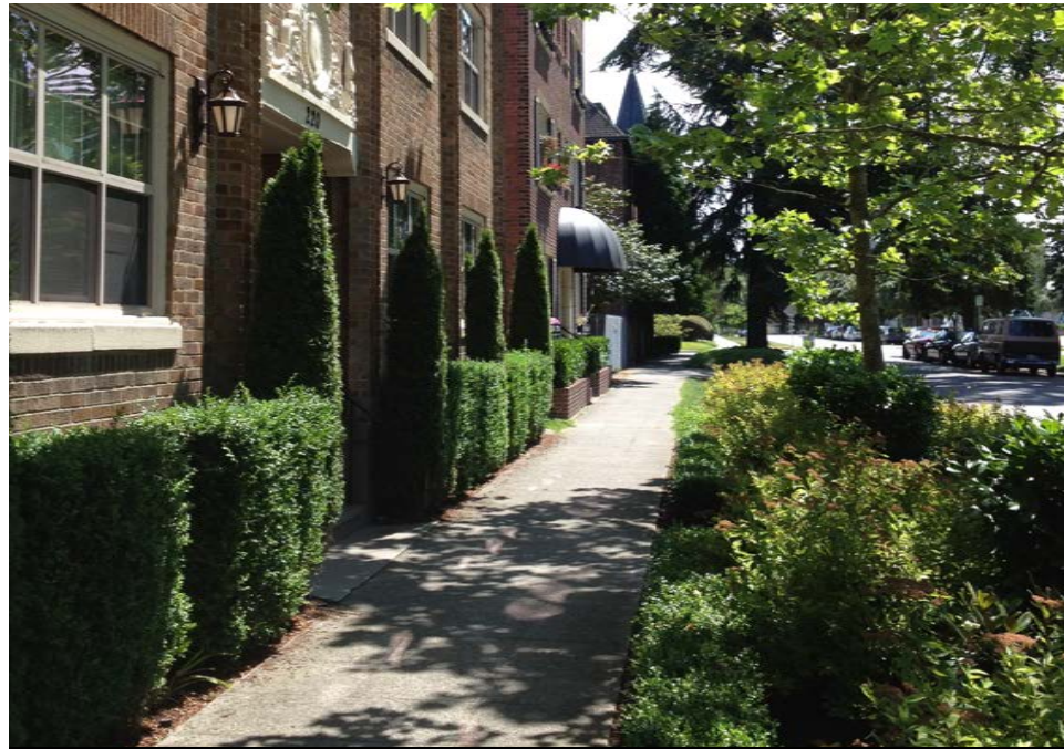
Design Cue: Well-defined street wall at Westland Manor & 214 16th Avenue East
