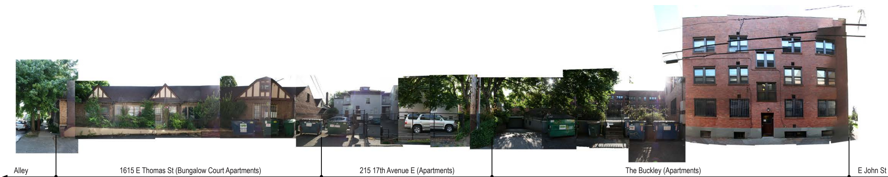
ALLEY PHOTO-MONTAGE LOOKING EAST
