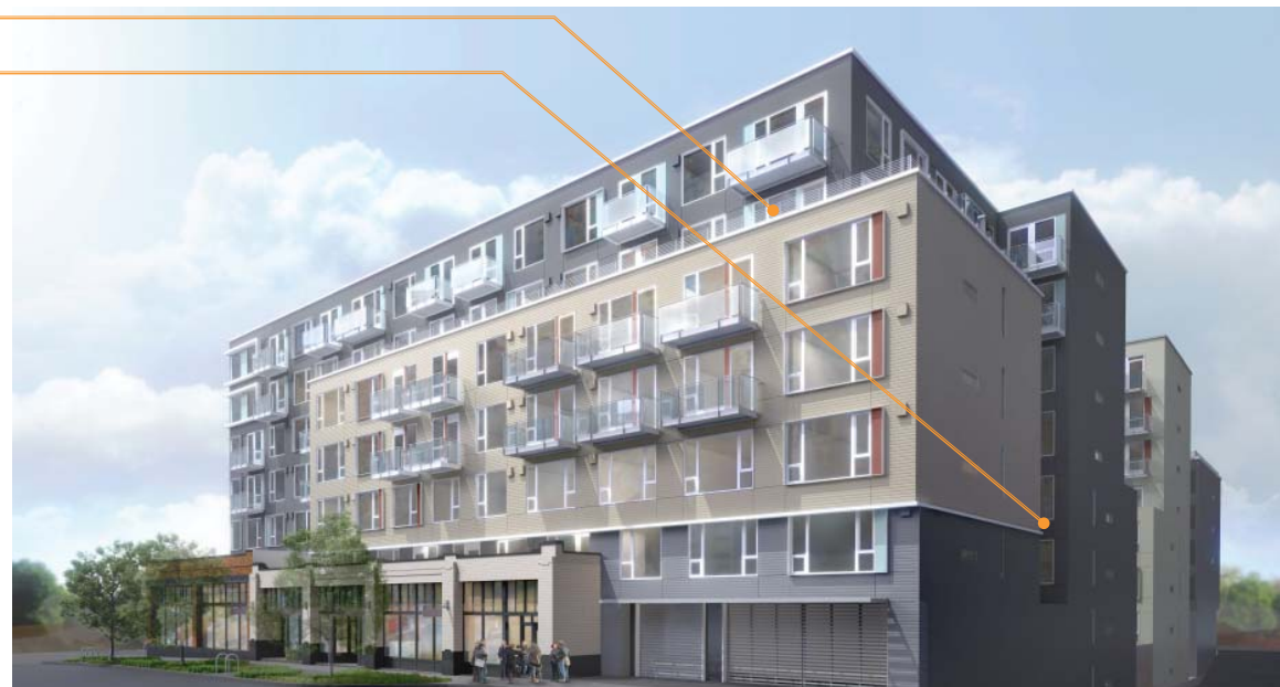
North Wall as Seen from 11th Ave
