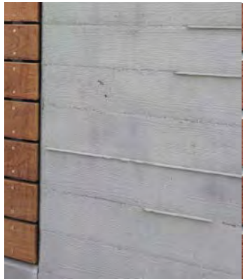
Board-formed concrete
