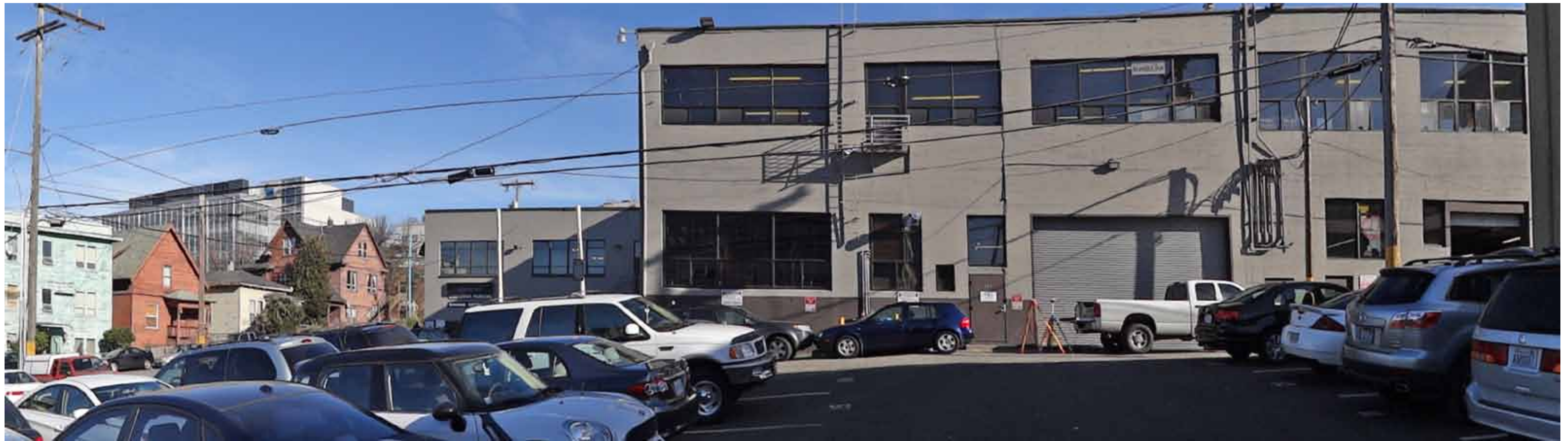
VIEW EAST TO SITE - ALONG ALLEY
