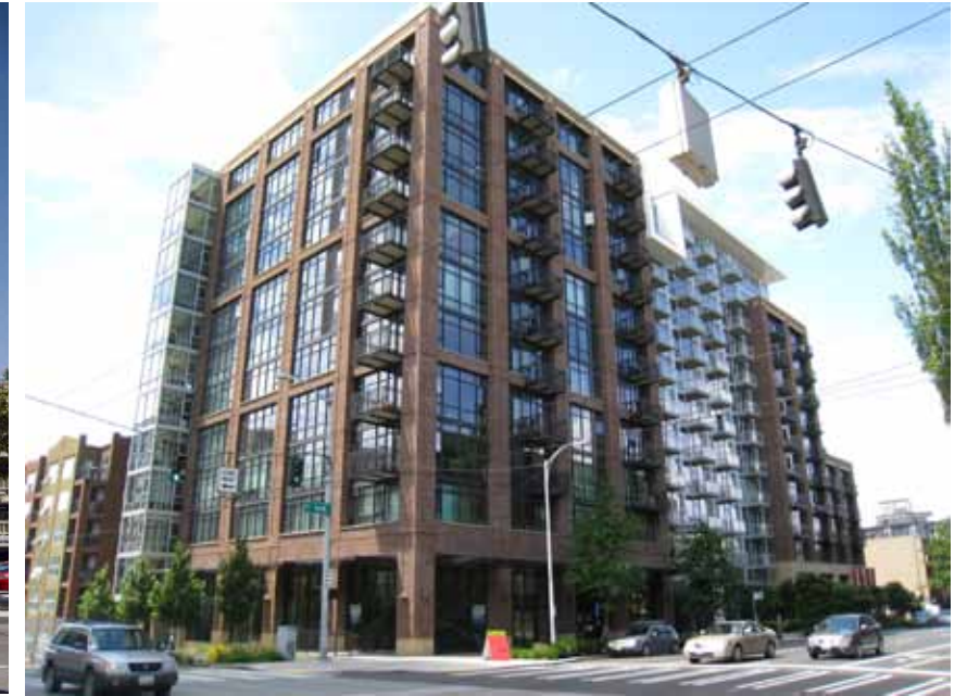
Large expanses of glazing for residential units.
