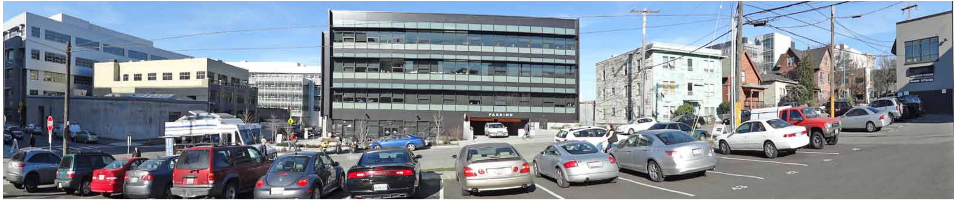
VIEW NORTH TO SITE - ALONG REPUBLICAN ST.
