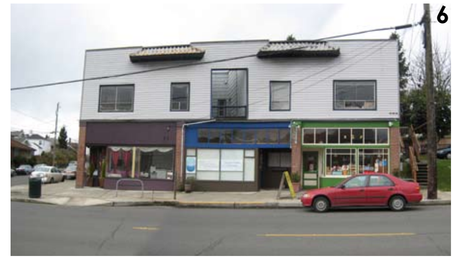
south end of site from 32nd Ave NW
