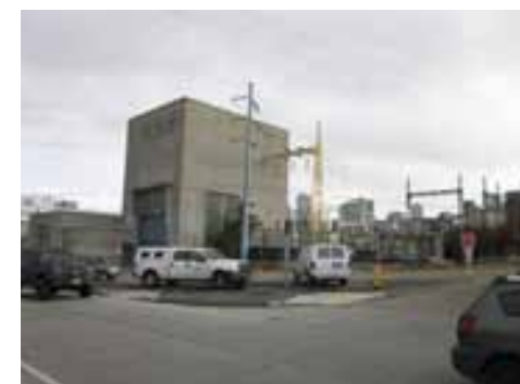
⑪ CITY LIGHT SUBSTATION
