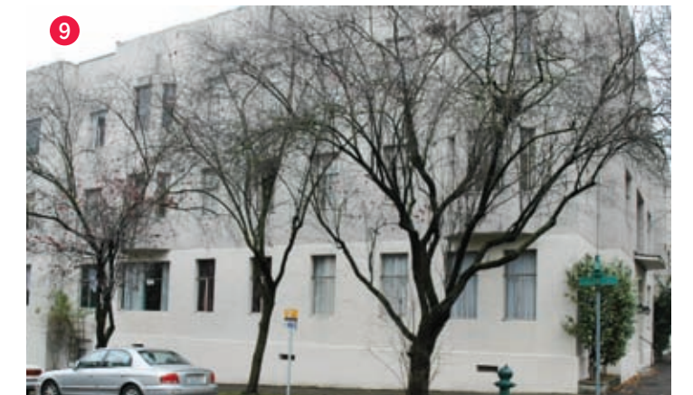
9 ST. PAUL APARTMENTS
