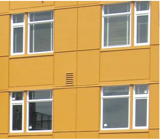
PANEL SIDING EXAMPLE FIBER CEMENT PANEL SIDING WITH REGLETS
