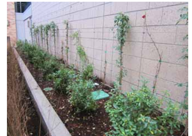
Vertical Planting Wall along Alley, delicate unclimbable cables
