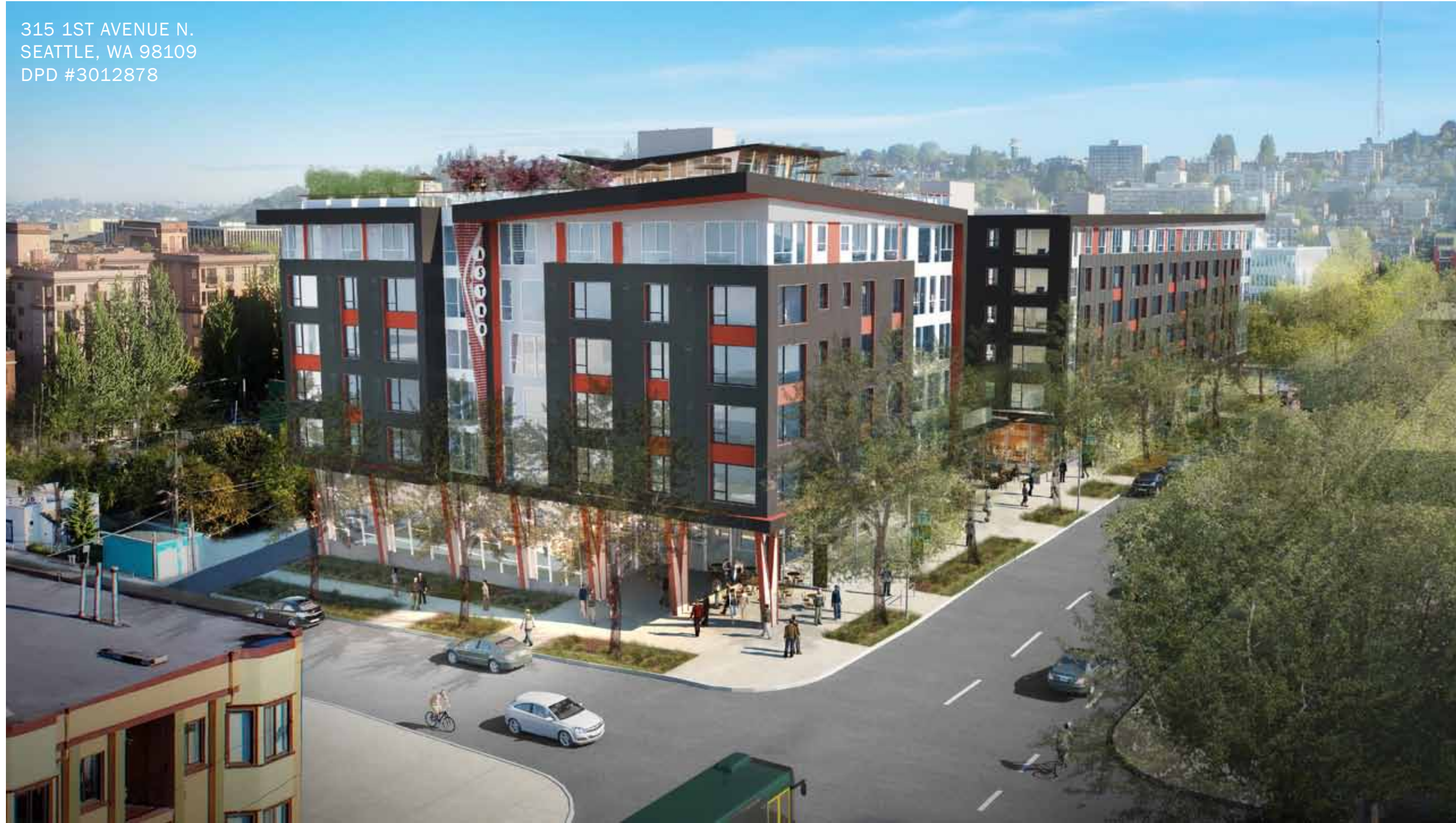
View of southeast corner at 315 1st Ave N.
