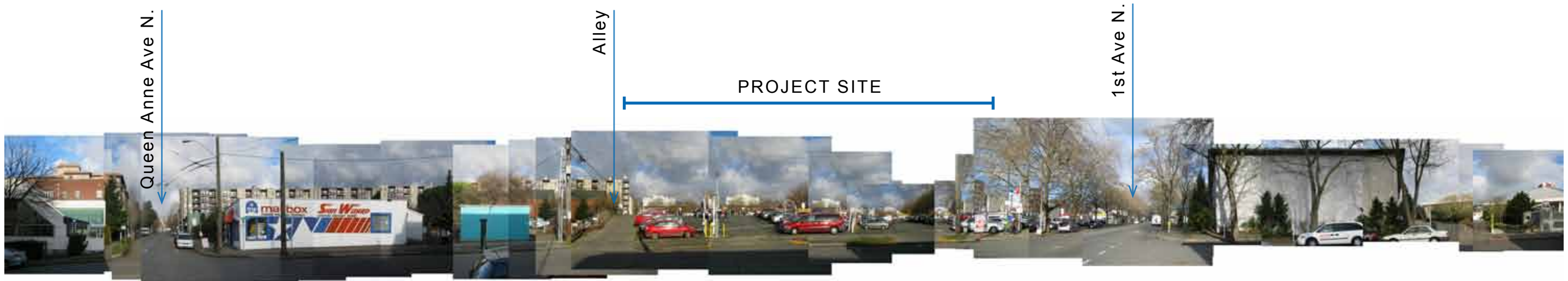
THOMAS STREET - Looking North (toward site)
