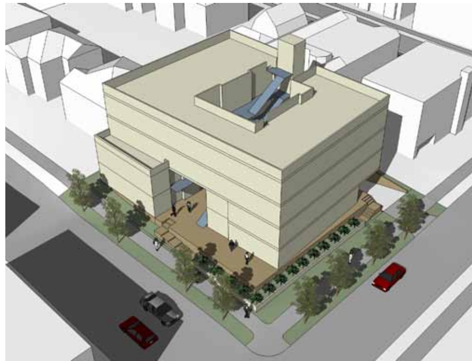
SW CORNER AERIAL VIEW
