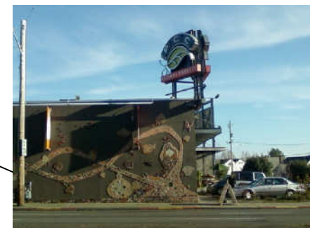
RECENT PCC RENOVATION
