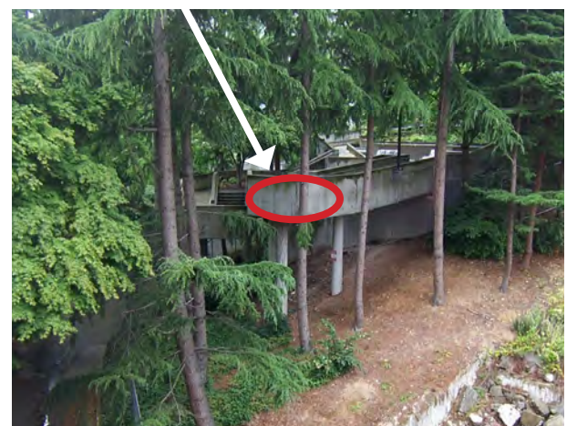
Point of Connection
