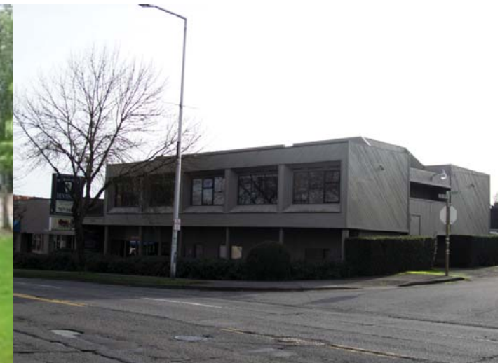
SW Roxbury Street
