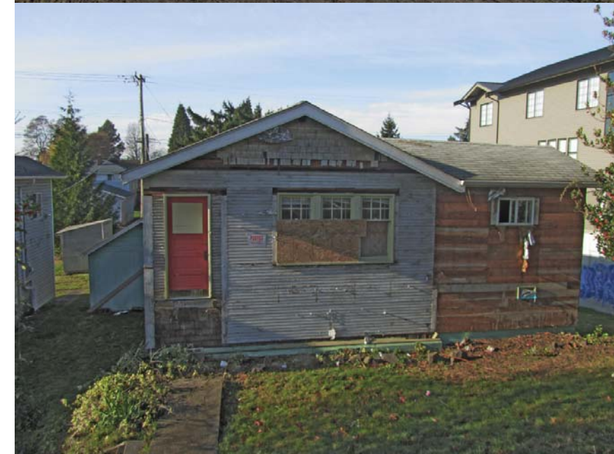
Existing structure on lot
