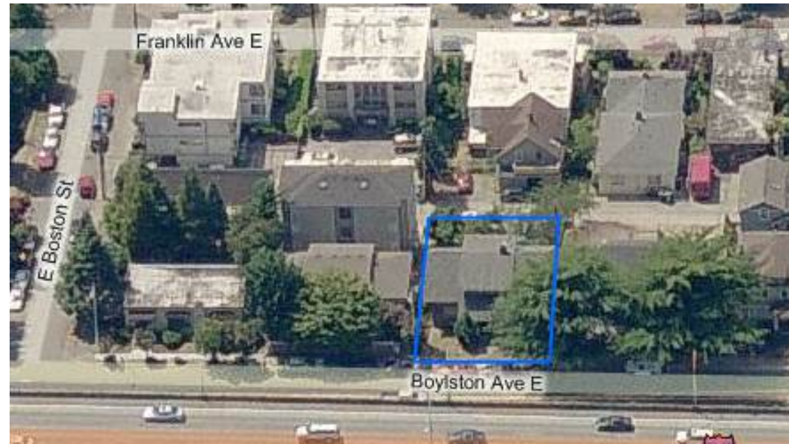
4 AERIAL LOOKING WEST
