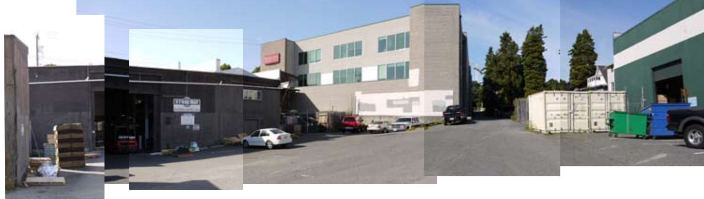
H LOOKING NORTH FROM MID-ALLEY AT CENTER OF SITE
