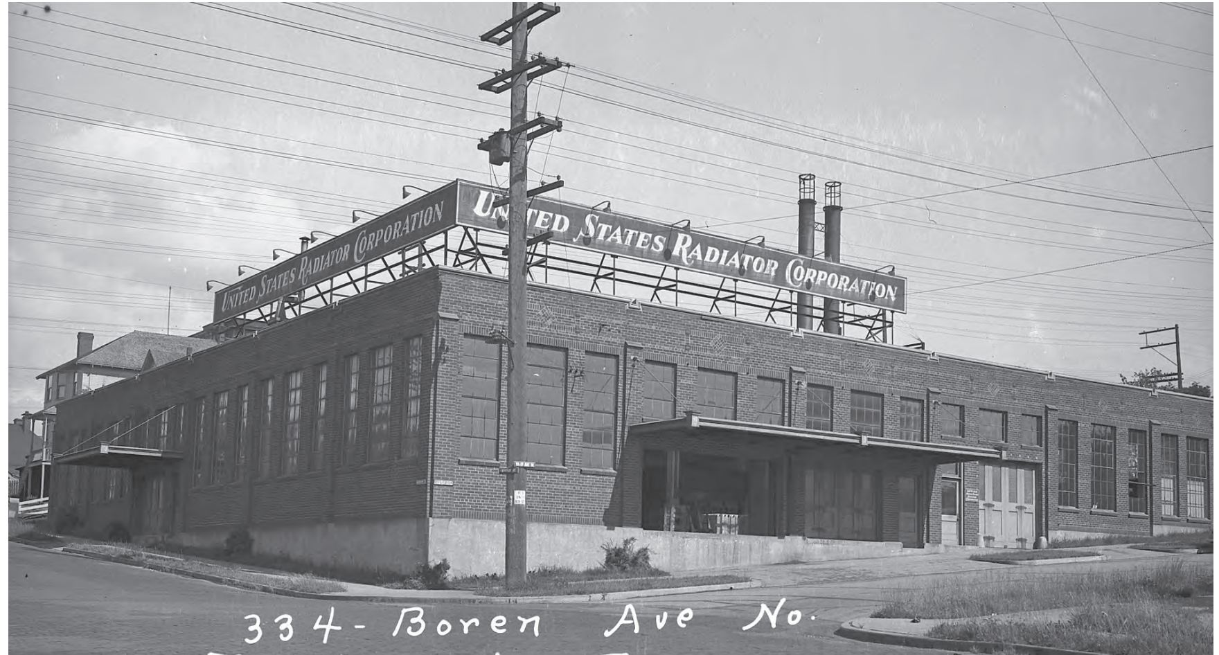
Boren Investment Building (1957 photograph)
