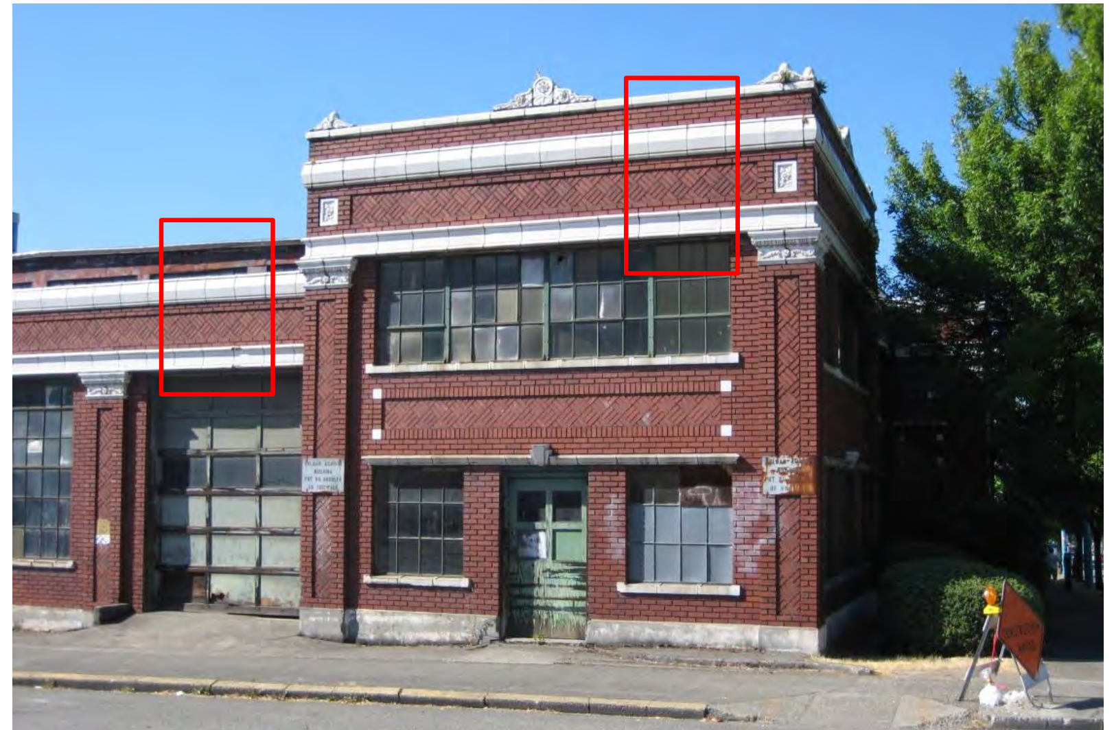
BRICK WALL SCALE AND TEXTURE
