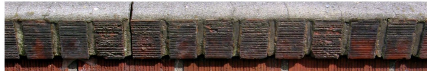
Boren Investment Building brick sill
