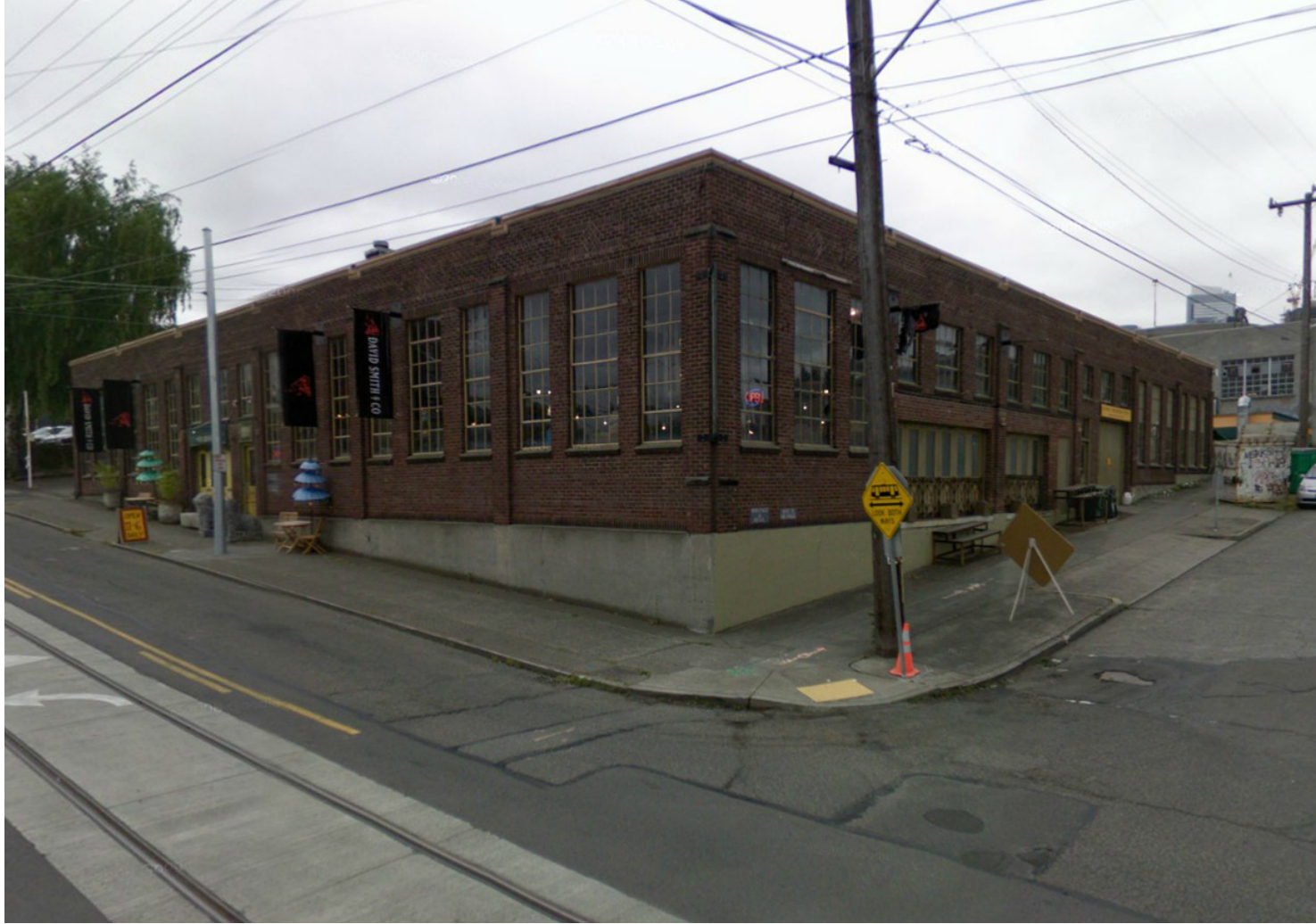
Boren Avenue North and Harrison Street
