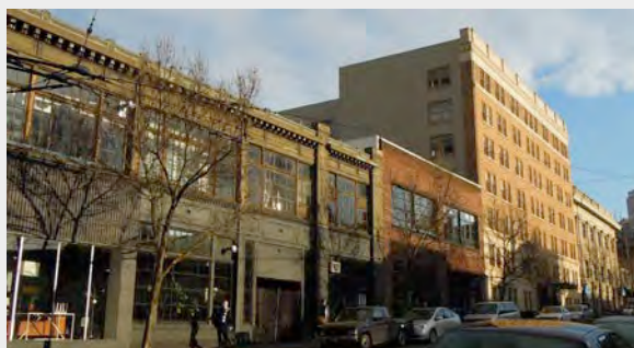
The New McDermott Building 1514 Bellevue Ave
