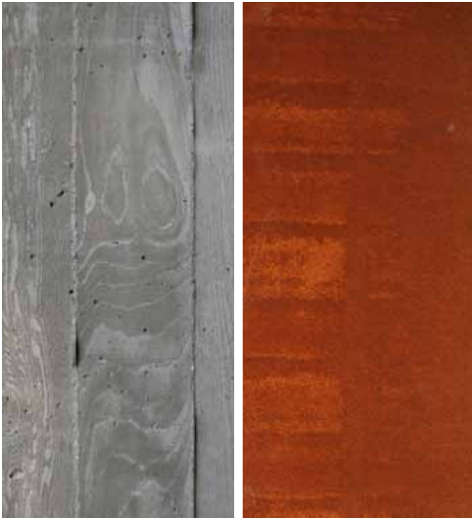
Steel (L) Concrete (L) Steel (R) Rusted Steel (R)
