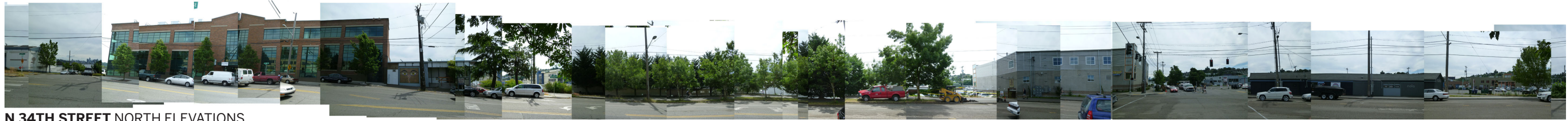
N 34TH STREET NORTH ELEVATIONS
