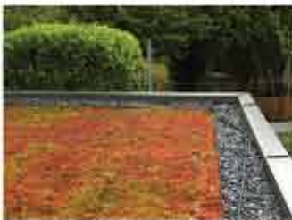
3' BALLAST BAND ALONG GREEN ROOF EDGE
