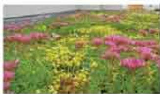
GREEN ROOF - SEDUM MAT
