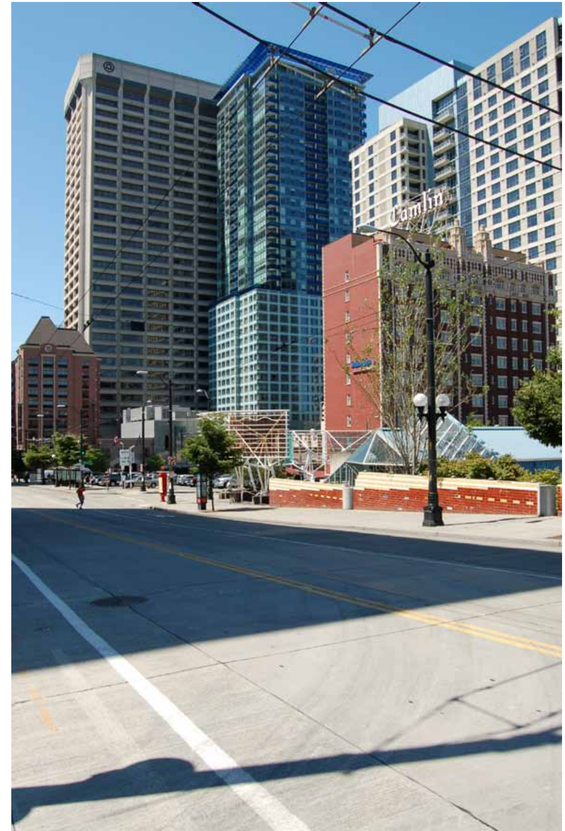
VIEW TOWARDS PROJECT SITE FROM PINE STREET LOOKING NW
