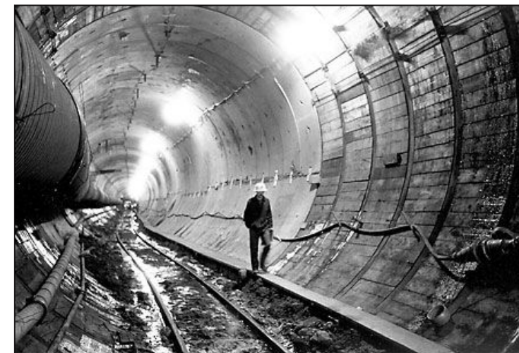
CONSTRUCTION OF METRO BUS TUNNEL UNDER THIRD AVE, 1988. CREDIT: SEATTLE P-I, CARY TOLMAN/SL
