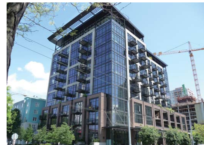
4 – Mosler Lofts (looking SouthEast)
