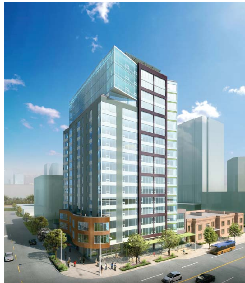
Alto Apartments - Under Construction
