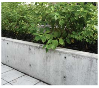
8 - Raised Concrete Planter
