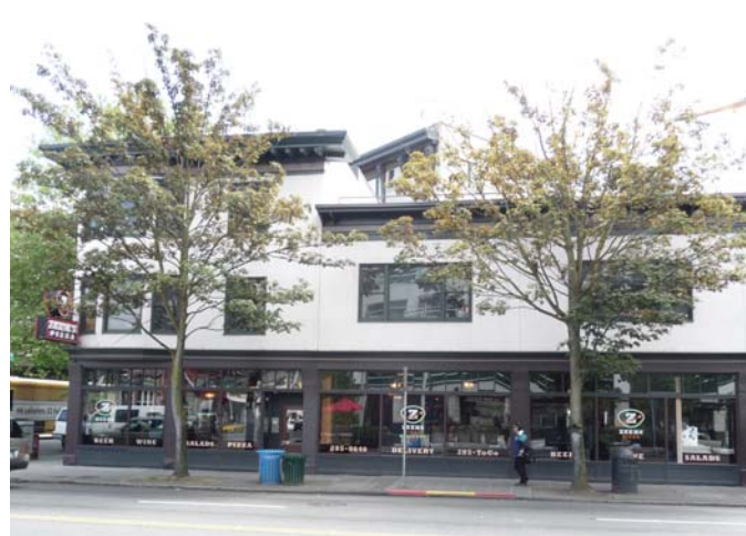
11 – Zeek's Pizza building (looking South)
