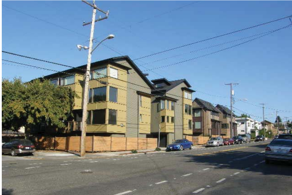
RESIDENTIAL CHARACTER NORTH OF SITE
