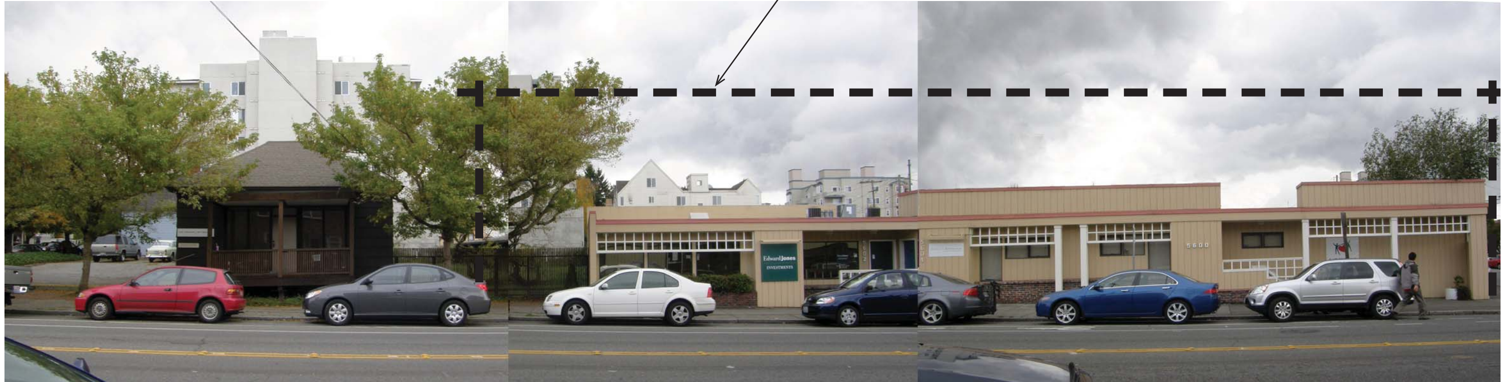
FROM 20TH AVENUE NW - LOOKING EAST
