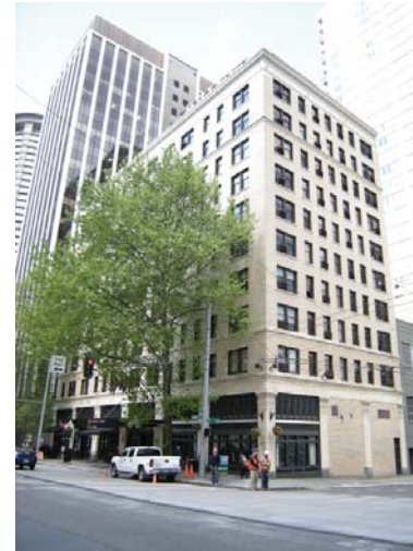
C: Hotel Max 620 Stewart Street Low-rise Urban Hotel Heavy Pedestrian traffic Punched openings
