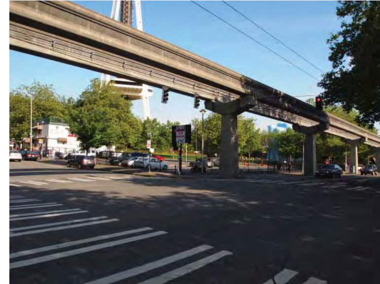
3. LOOKING WEST (ACROSS 5TH AVE N) AT SITE
