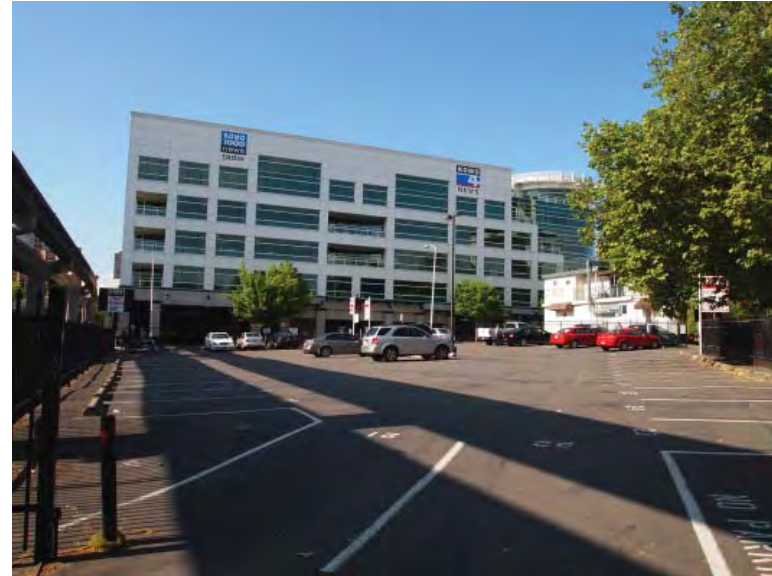
2. LOOKING SOUTH (ACROSS SITE) AT FISCHER PLAZA
