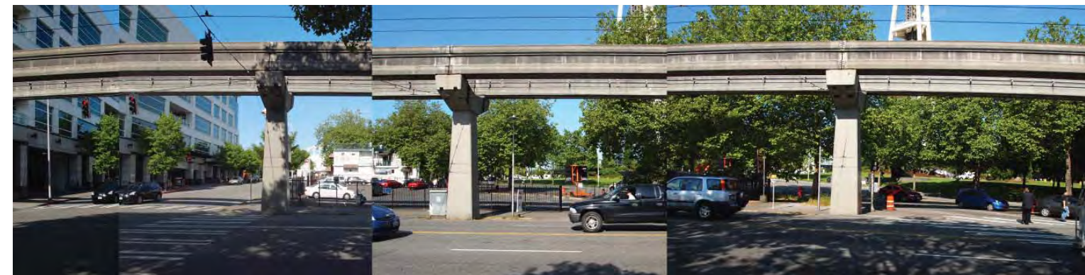
LOOKING WEST (ACROSS 5TH AVE N) AT SITE
