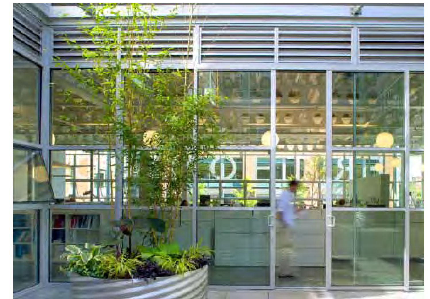
ALUMINUM STOREFRONT WINDOWS AT COMMERCIAL SPACE FINISH: CLEAR ANODIZED
