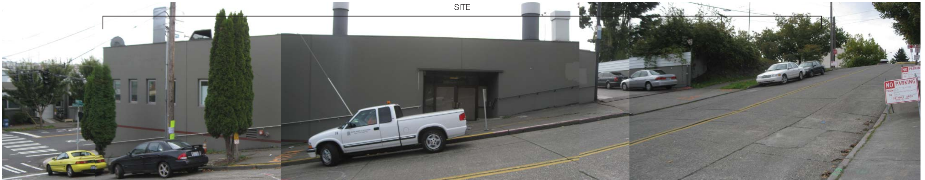
Site view from Aloha St.
