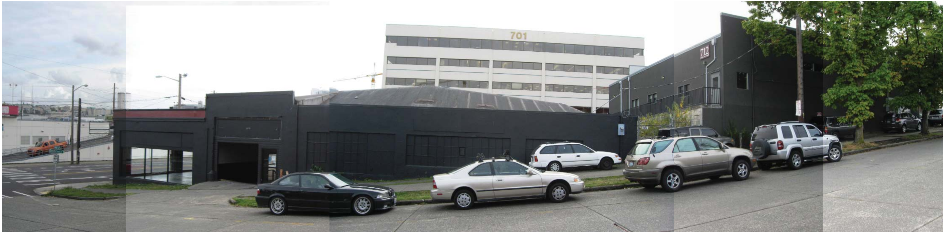
View South from Valley St.
