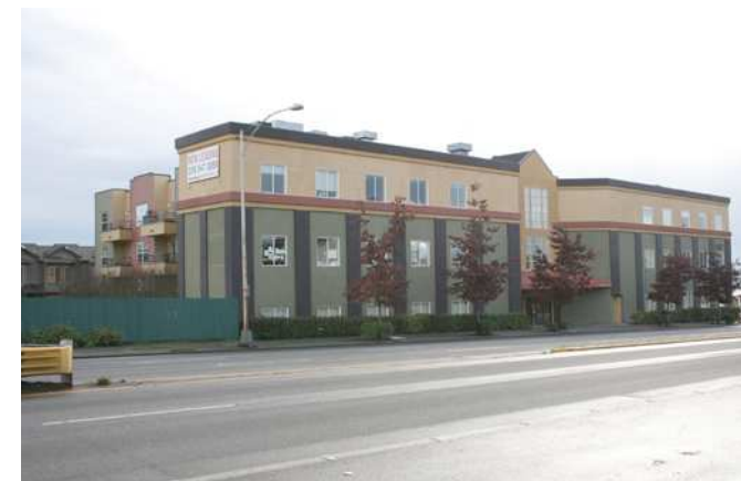
12 - Looking Southeast on Aurora
