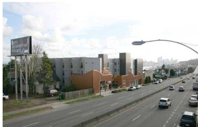
10 - Looking Southeast on Aurora
