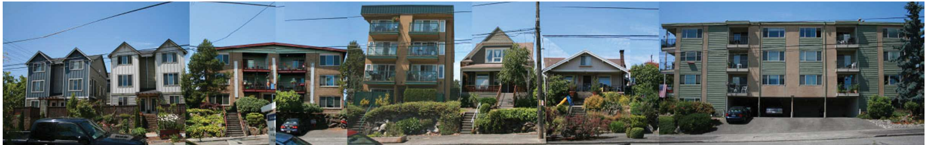
9 - Looking West across Whitman Ave N
