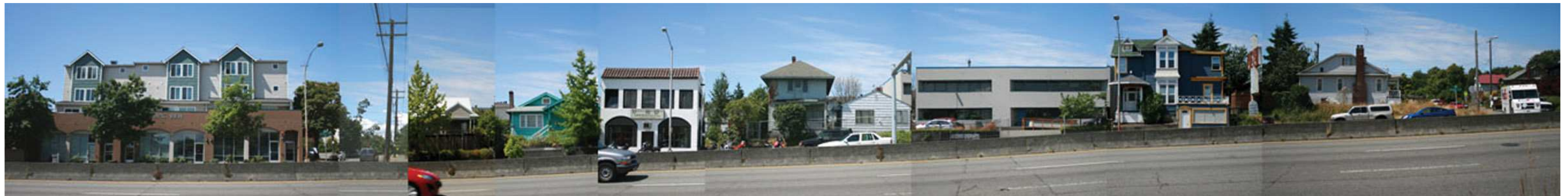
1 - Looking West from the Site
