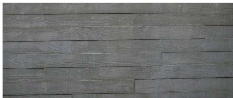
④ BOARD FORMED CONCRETE
