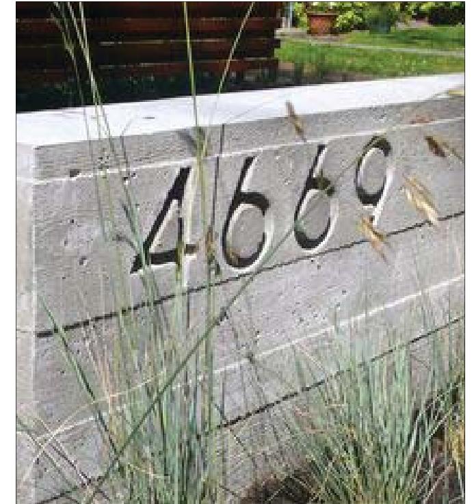
⑰ BOARD FORMED CONCRETE SIGNAGE
