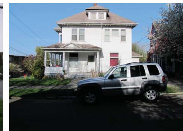
④ VIEW FROM 11TH AVE E
