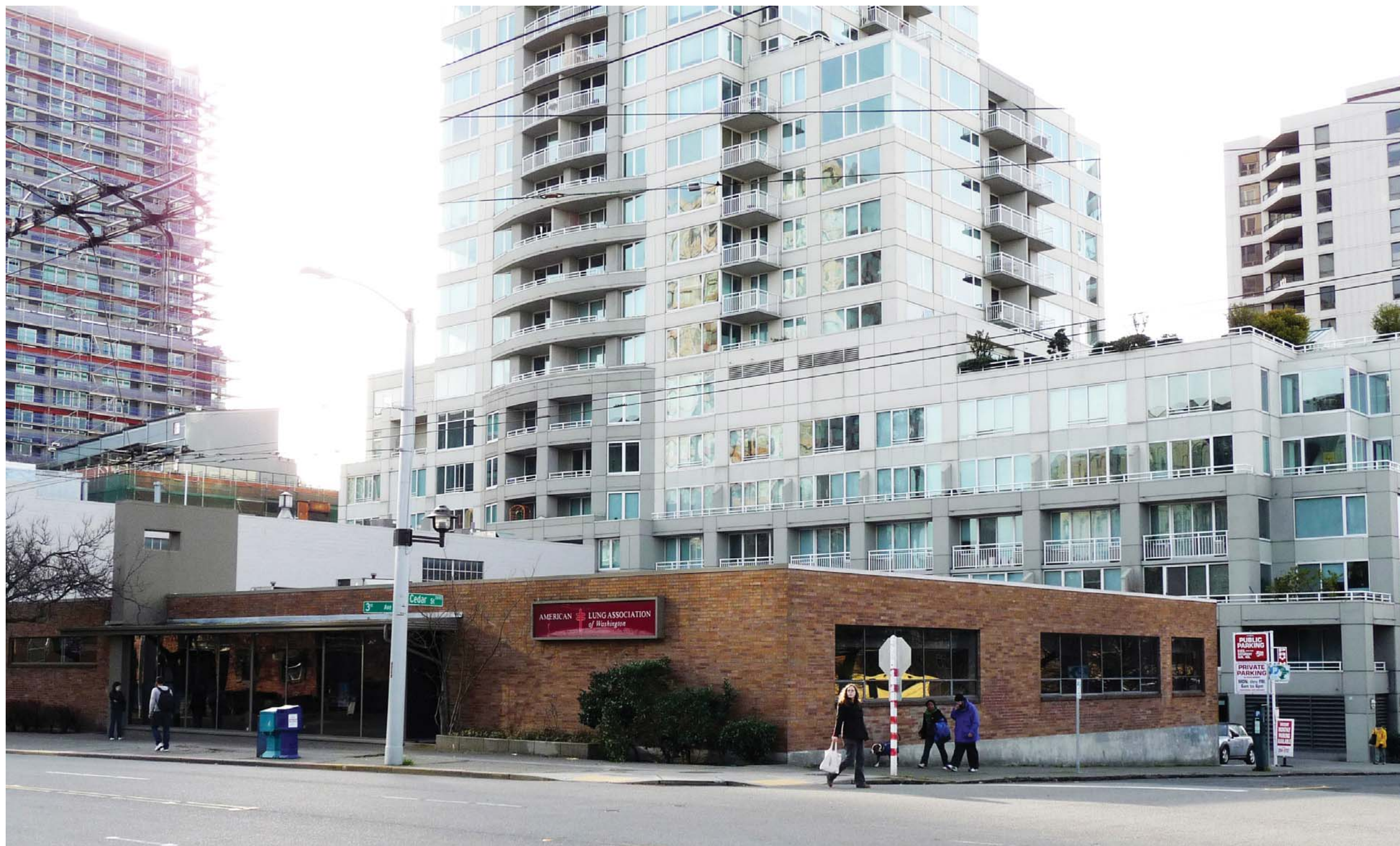
The proposed project's alley massing strategies are in response to the alley-facing units of the adjacent Seattle Heights building.
