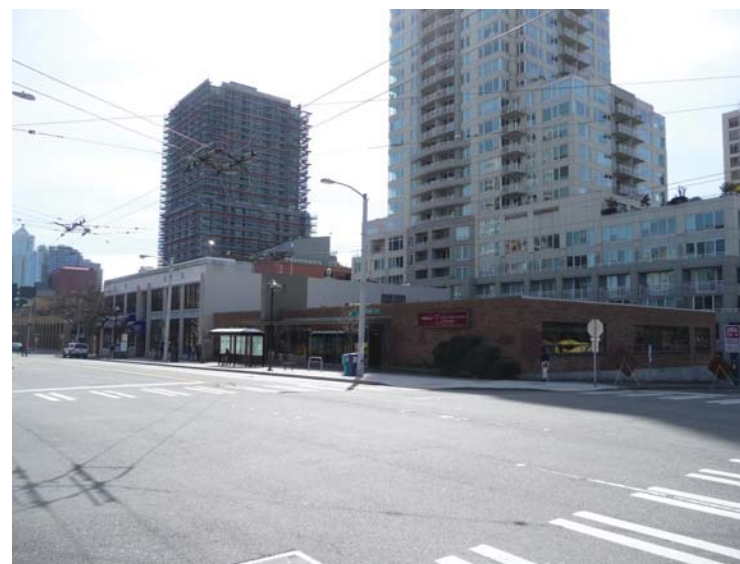
1 - 2612 3rd Avenue (project site) looking SouthWest
