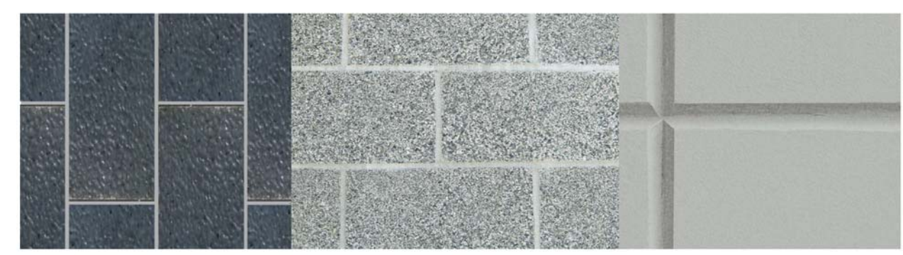
Glazed Tile Groundface CMU Painted and Scored Concrete
