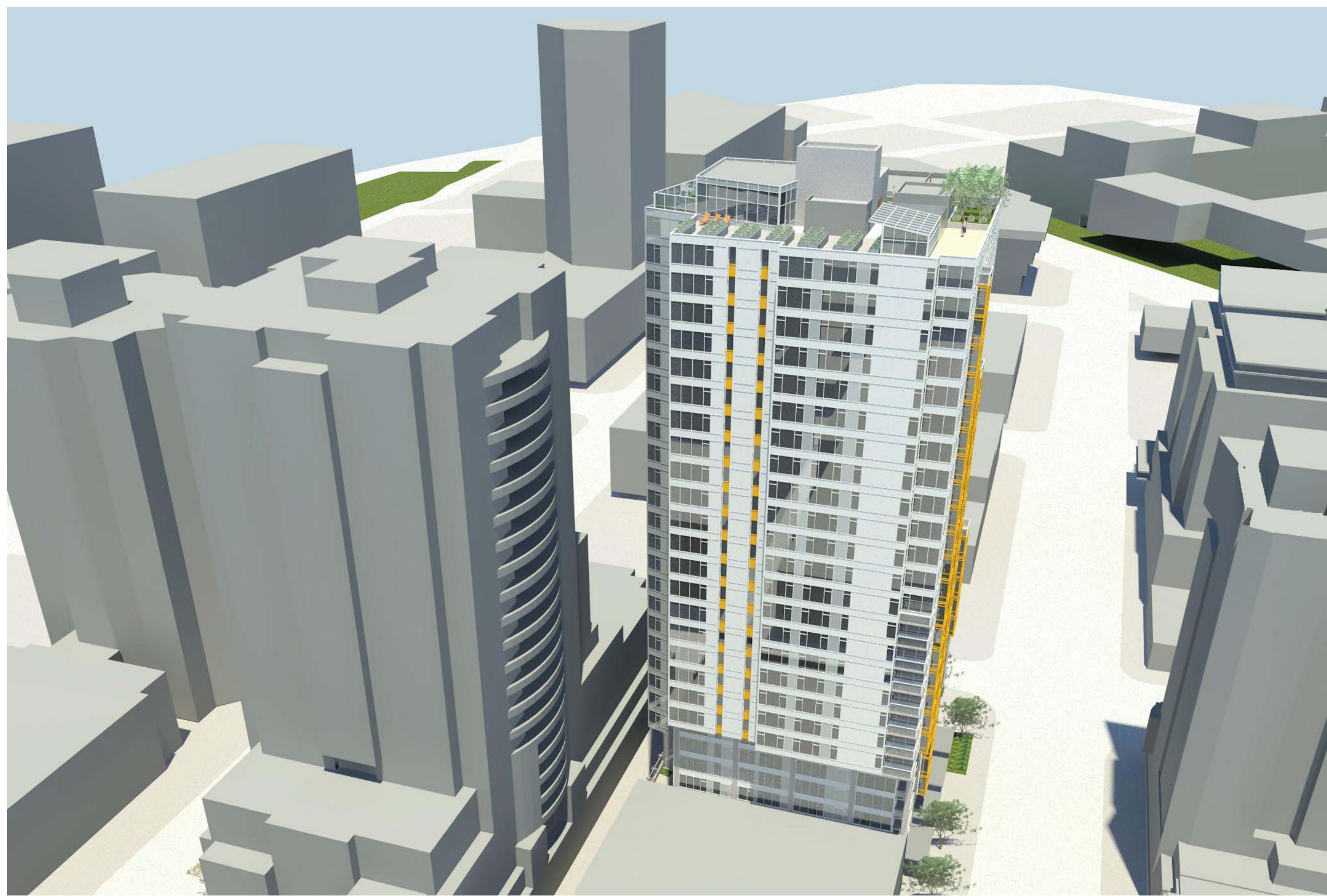
Context View – South
