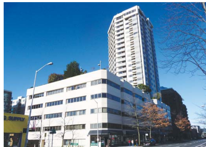
9 – Bay Vista Tower (looking West)
