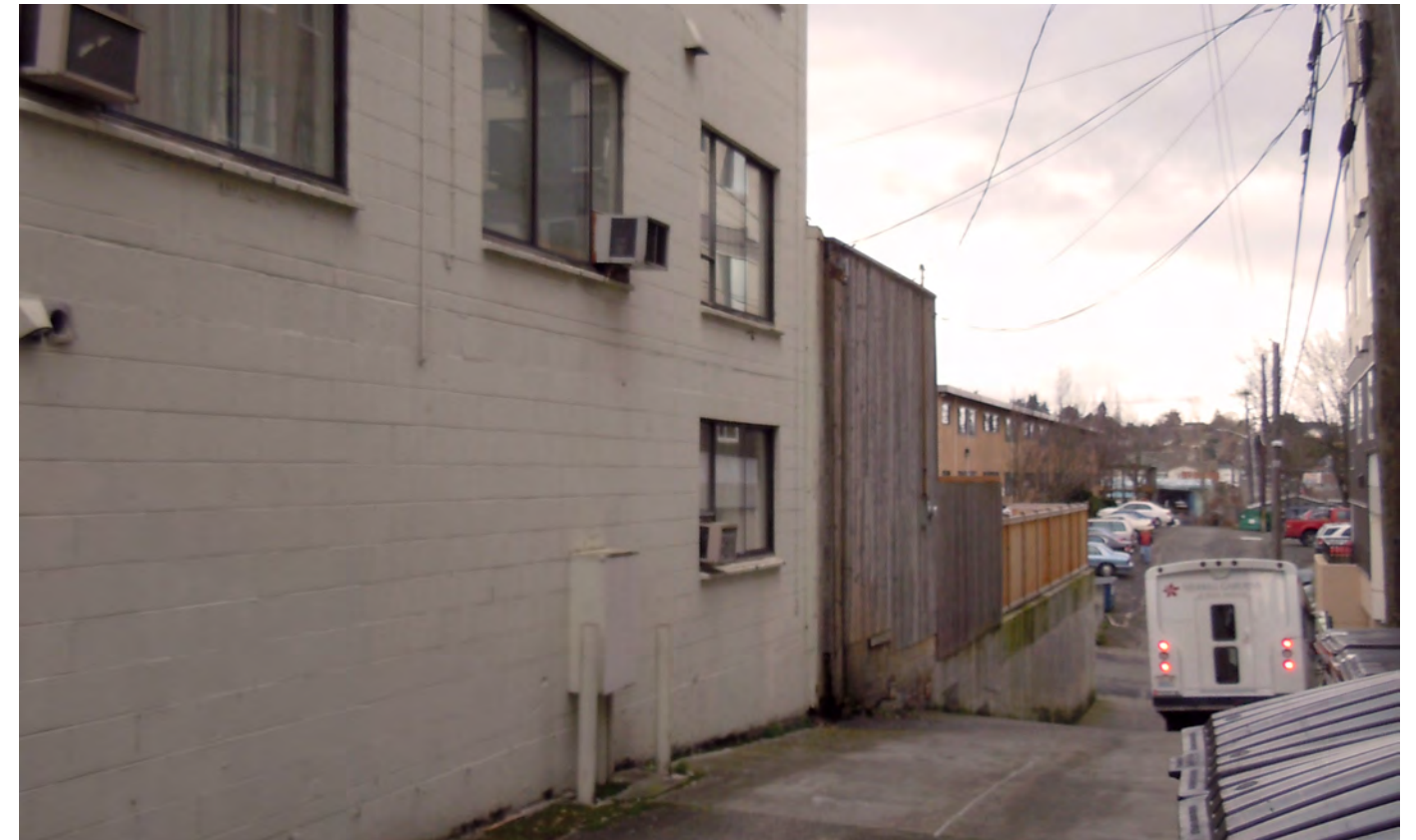
VIEW OF SITE FROM ALLEY
