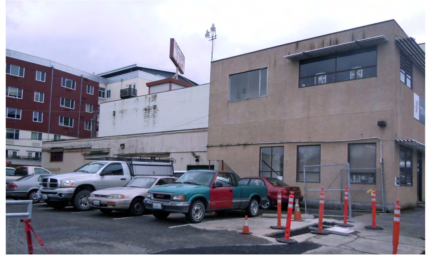
VIEW OF ADJACENT BUILDING TO SOUTH (TAN BUILDING IN FOREGROUND TO BE DEMOLISHED)
