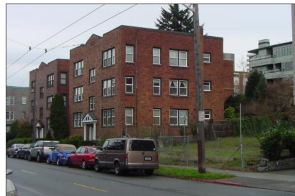
VIEW OF ADJACENT BUILDING TO NORTH
