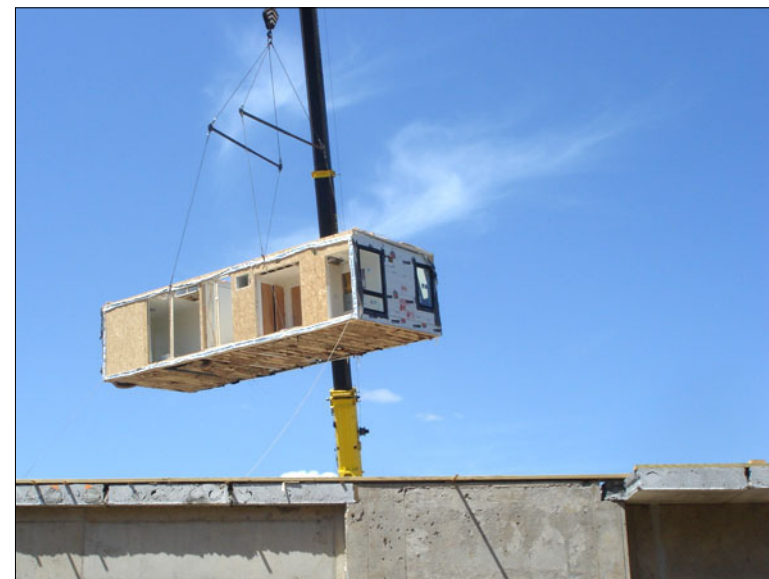
ASSEMBLY OF MODULES ON SITE
