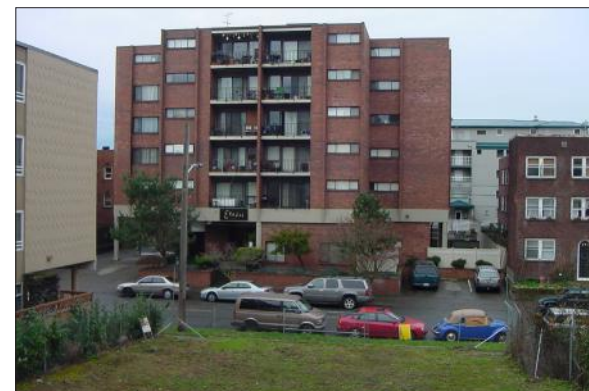
VIEW OF SITE FROM ALLEY, LOOKING WEST
