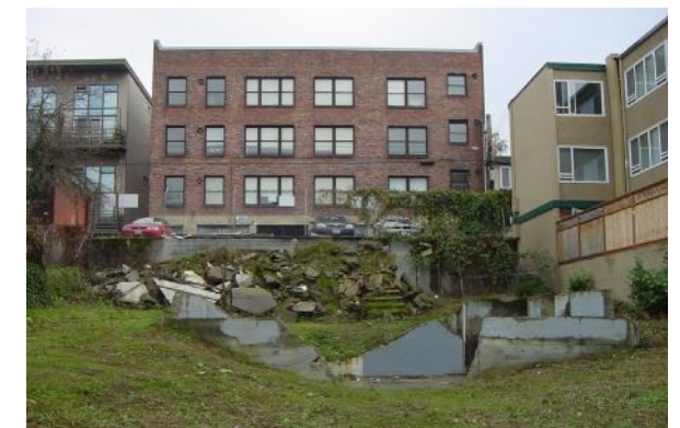
VIEW OF SITE FROM BELLEVUE AVE LOOKING EAST
