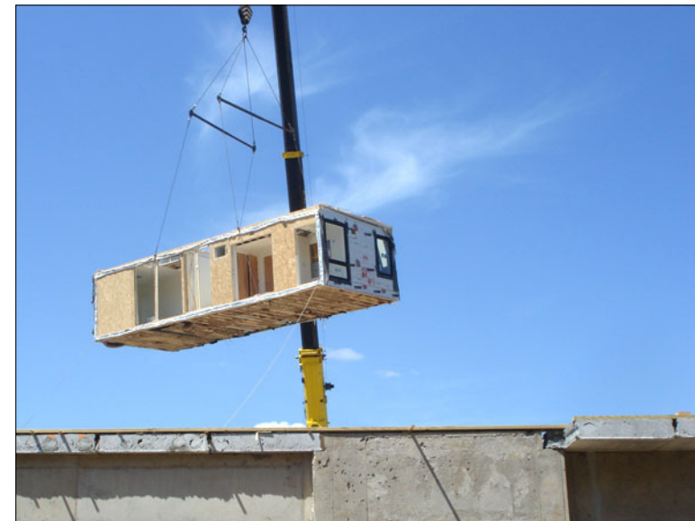
ASSEMBLY OF MODULES ON SITE
