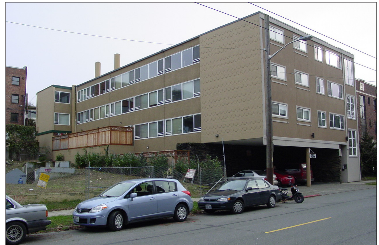
VIEW OF ADJACENT BUILDING TO SOUTH
