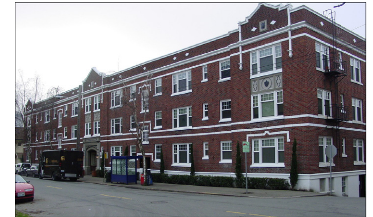
EXISTING BUILDINGS IN THE NEIGHBORHOOD WITH MINIMAL OR NO SETBACKS
