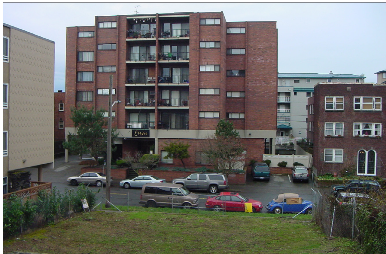
VIEW OF SITE FROM ALLEY
